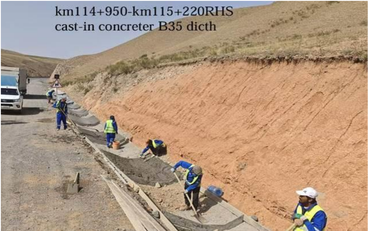
Figure 11: Cast-in concrete B35 ditch, km 114+950 – km 115+220 RHS.
