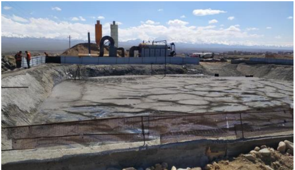
Figure 23: Bitumen pit at the production site (km 148+630).
