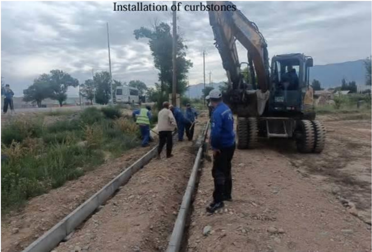
Figure 5: Installation of curbstones, km 143+114 – km 143+615, LHS.
