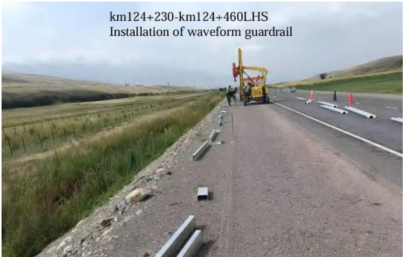
Figure 7: Installation of waveform guardrail, km 124+230 – km 124+460, LHS.
