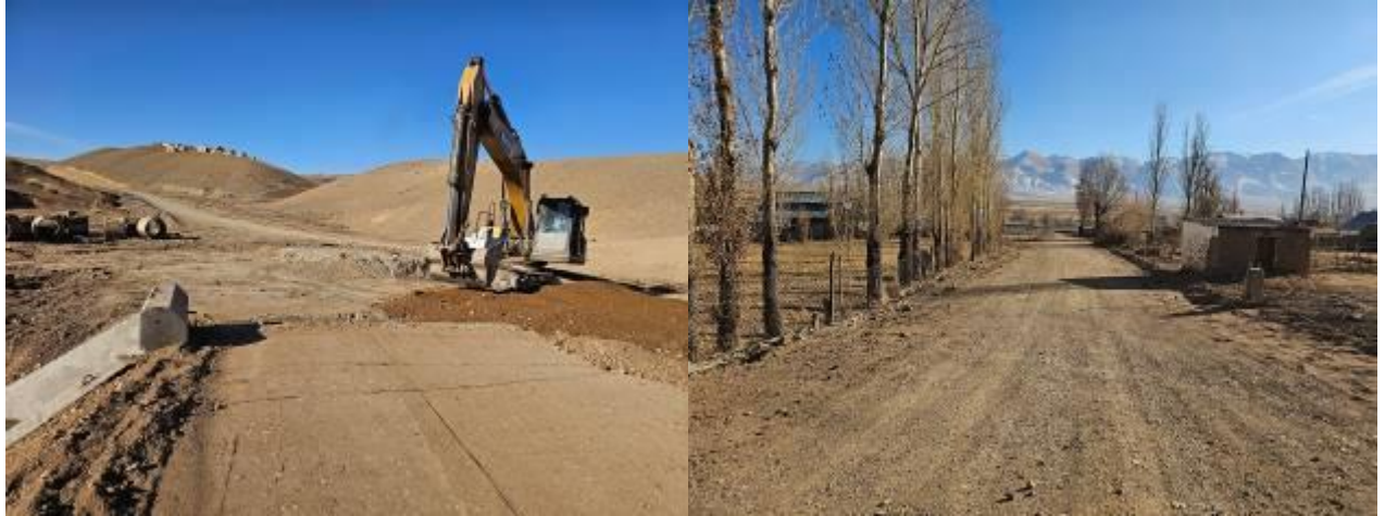
Figure 15: Access road to Lama Village (5.801 km)
