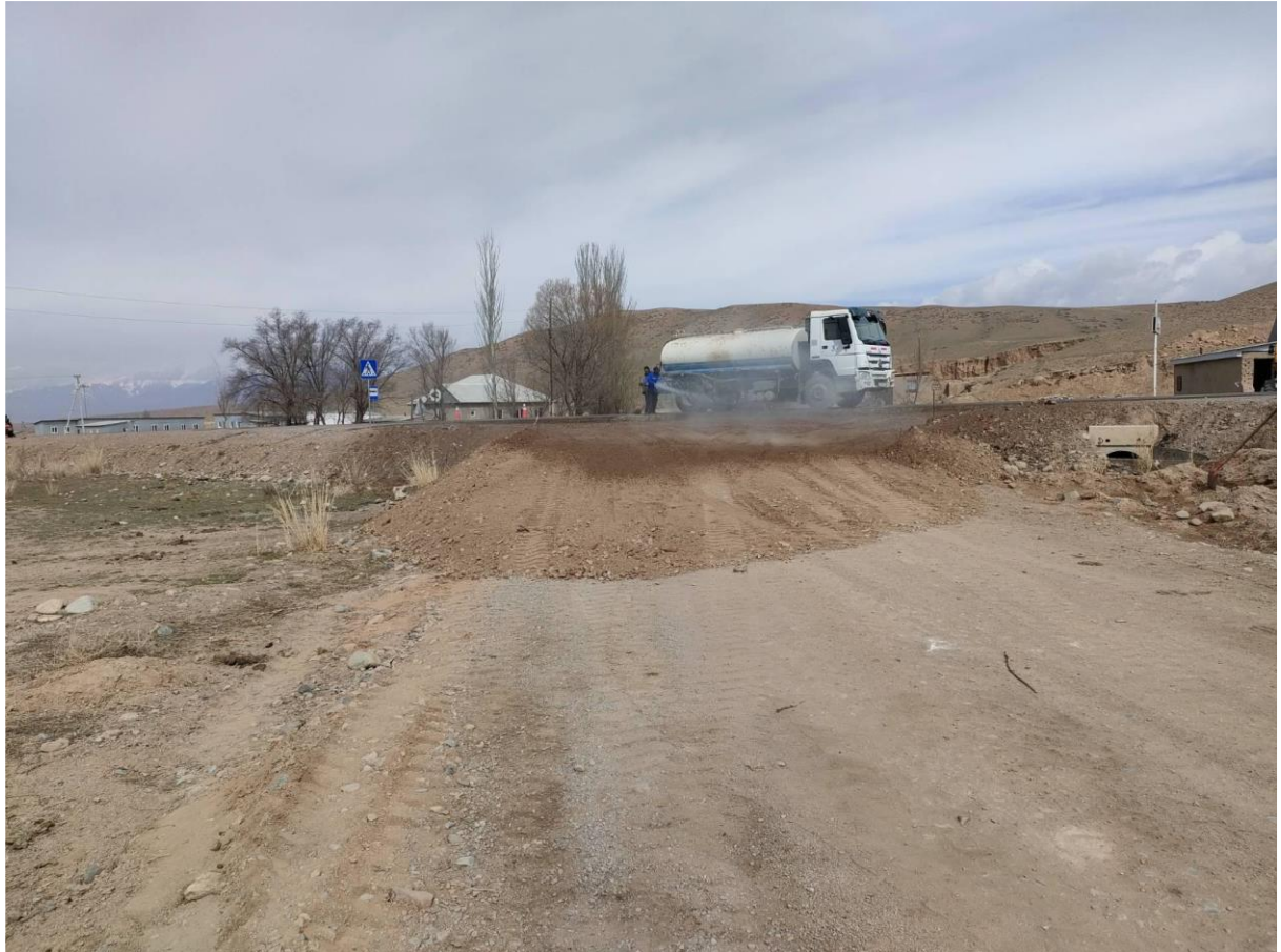
Figure 18: Dust suppression during intersection earthwork construction on km 137+062 (LHS).
