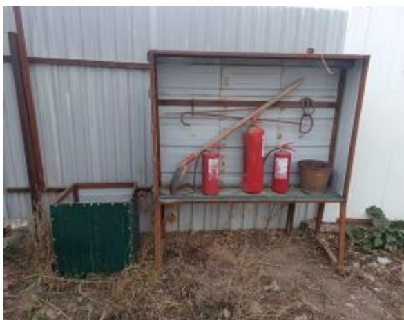
Figure 35: Equipped fire safety boards
