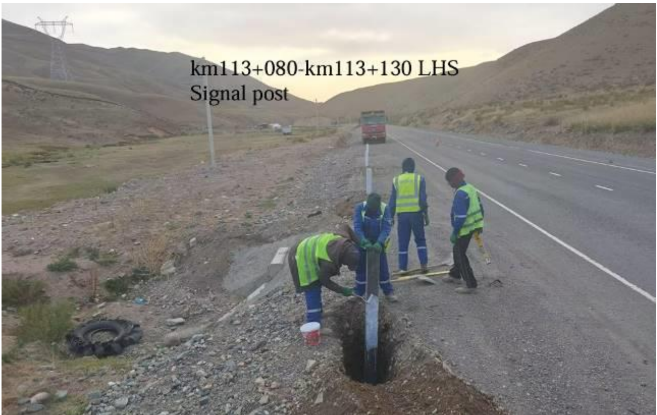
Figure 12: Signal posts installation, km113+080 - km113+130 LHS.
