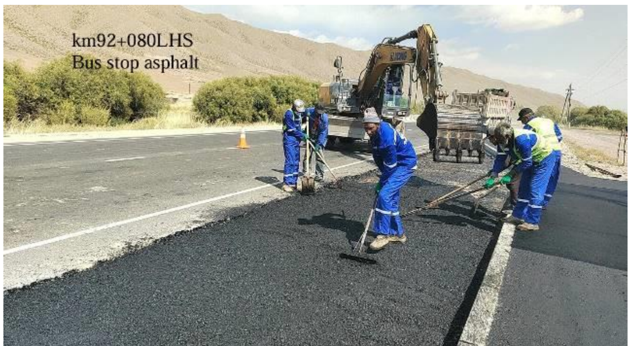
Figure 8: Asphaltting of a bus stop, km 92+080, LHS.
