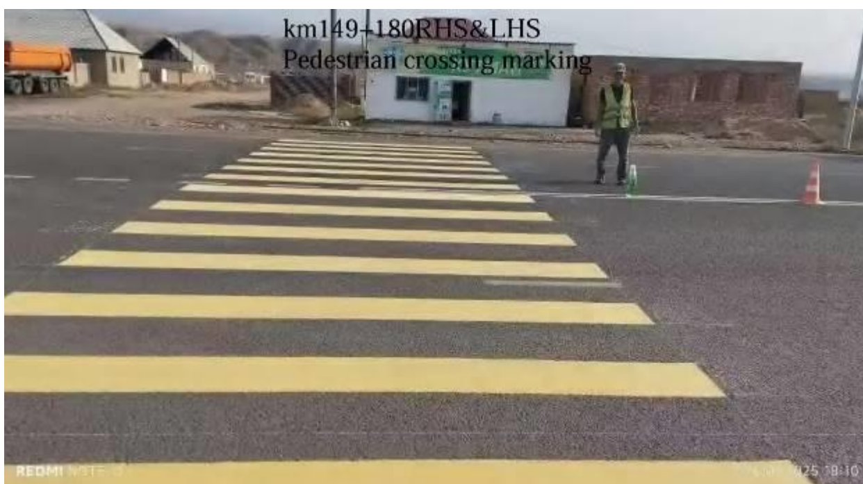
Figure 4: Pedestrian crossing marking, km 149+180
