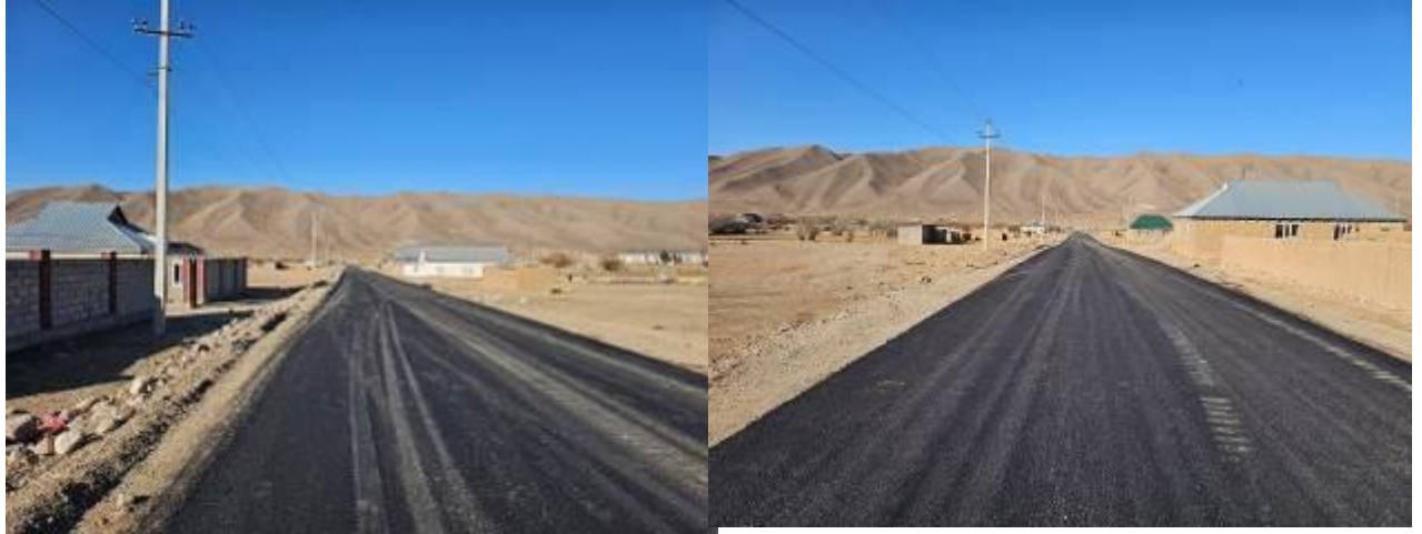
Figure 16: Access road to Ak-Chyi Village from the project road (0.545 km)
