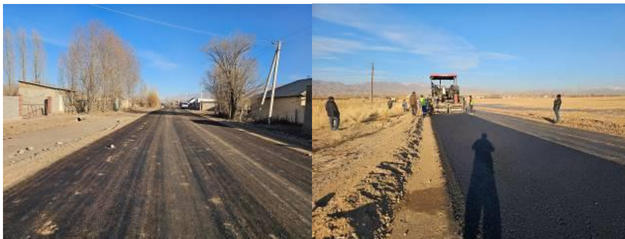
Figure 13: Access road Kuyruchuk – Shilvili (1.562 km)
